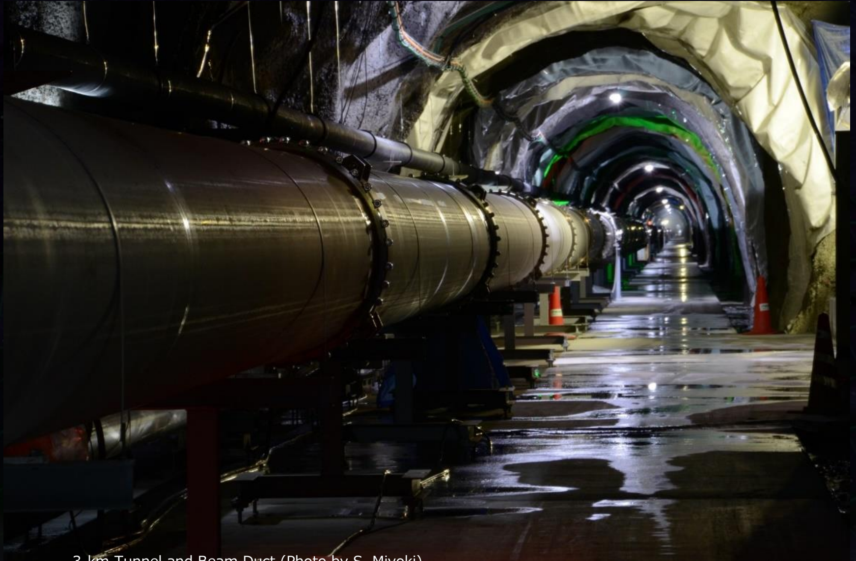
3-km Tunnel and Beam Duct (Photo by S. Miyoki)
