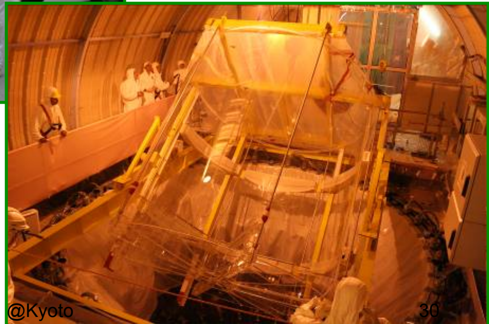
Acrylic tank installation (8~9/2009)
